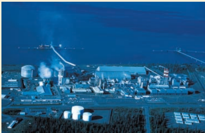
▲ Today, ammonia is produced on an industrial scale in plants like this one.
